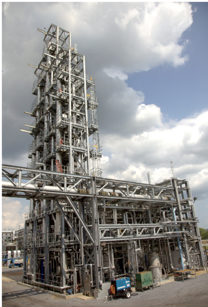
FIGURE 3.6 Conventional amine solvent plant for CO 2 separation at the National Carbon Capture Center in Wilsonville, Alabama. This is a demonstration plant that bridges technologies from the bench-scale to pilot scale, and the absorber unit that is currently in place captures 3,650 tCO 2 per year. In contrast to the air contactor used for extremely dilute air capture, this flue gas contactor (absorption column) can be tall for increased CO 2 separation due to the inherent driving force of the flue gas stream. This image provides an example for dimensional comparison to the DAC plant in Figure 3.5, not a comparison of scale as the annual removal rate by the National Carbon Capture Center is small since it is for demonstration purposes only. SOURCE: Courtesy of Frank Morton, Business Development Manager of the National Carbon Capture Center, Southern Company.
